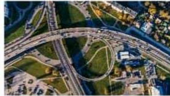
10 LANE - AHMEDABAD TO DHOLERA EXPRESSWAY
