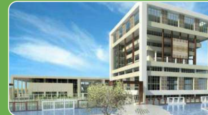
DHOLERA ABCD BUILDING
