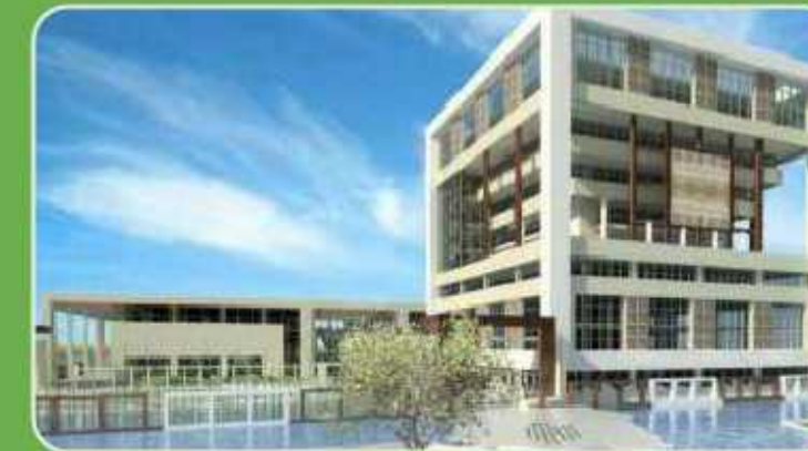
DHOLERA ABCD BUILDING
