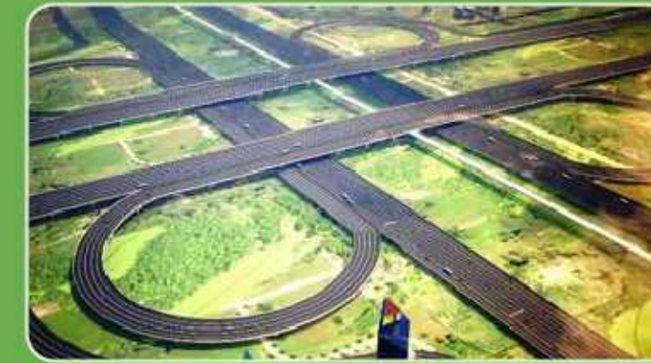
250 M WIDE 6 LANE AHMEDABAD-DHOLERA EXPRESS WAY
